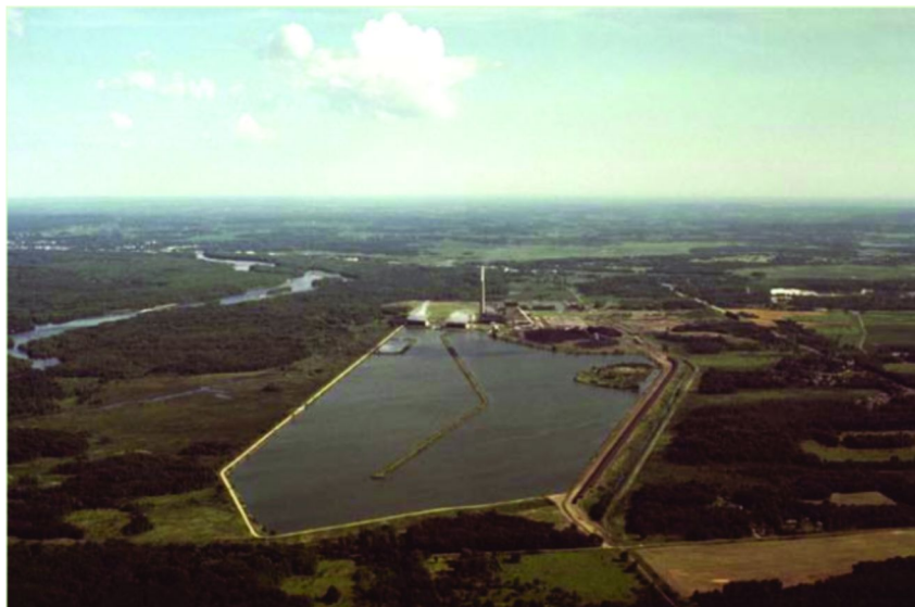
Figure 13. The Wisconsin Power and Light Columbia Plant uses vast quantities of water per hour, and circulates that water in a large cooling lake located immediately next to the plant. Locations like this may present an opportunity for low cost retrofitting for algal carbon capture. (Image from Louis J. Maher, Jr., University of Wisconsin)
